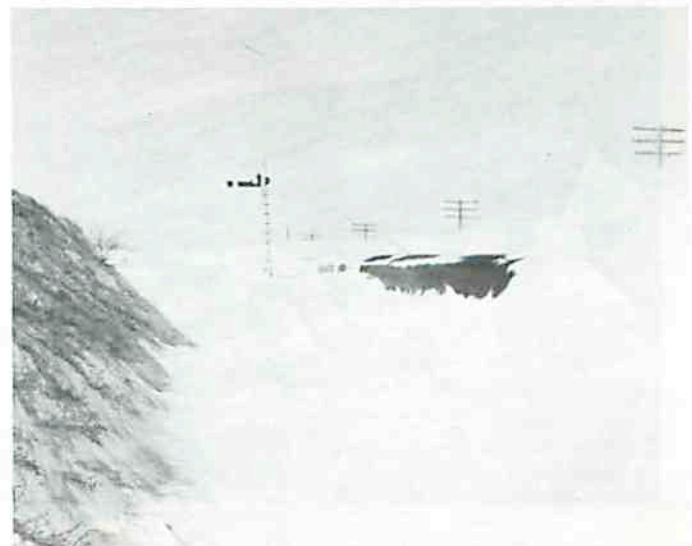
NPRR #1 - blocked near North Almont - March 1966.
